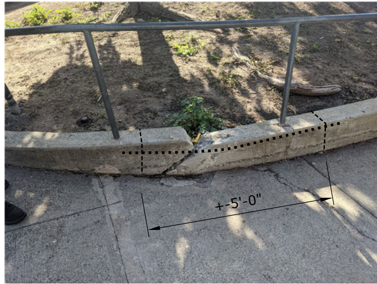
LOCATION: TOP OF RAMP AT AREA 5. REMOVE AND REPLACE (E) CURB. #4 REBAR DOWELED IN 12" MIN.
