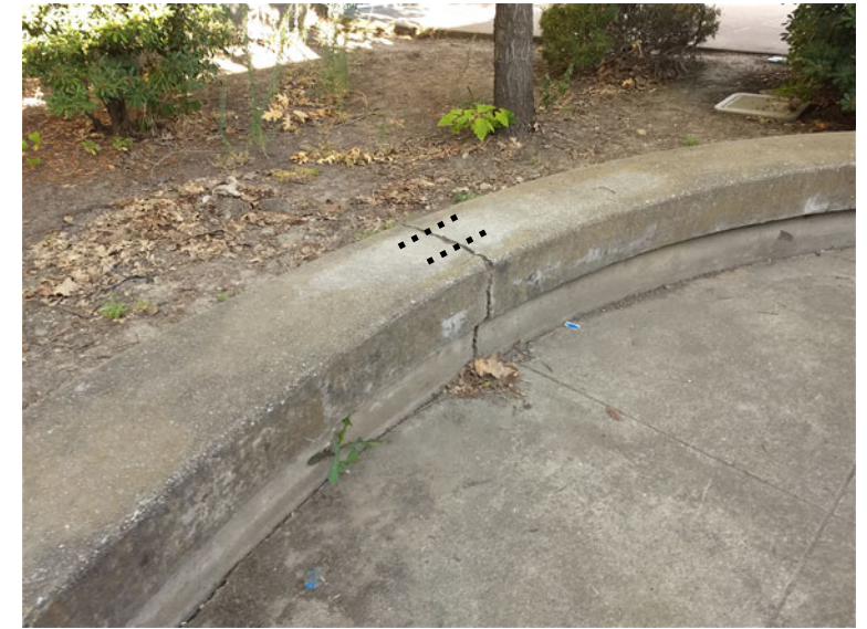
LOCATION: COURTYARD BETWEEN POD B AND POD C. REPAIR (1) CRACK. SAWCUT 3" DEEP SLOTS TO INSERT #4 REBAR, 12" LONG. (2) EA. SIDE.
