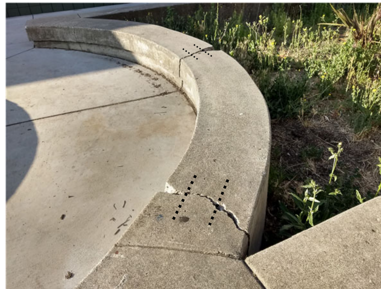
LOCATION: COURTYARD BETWEEN POD B AND POD C. REPAIR (2) CRACKS. SAWCUT 3" DEEP SLOTS TO INSERT #4 REBAR, 12" LONG. (2) EA. SIDE.
