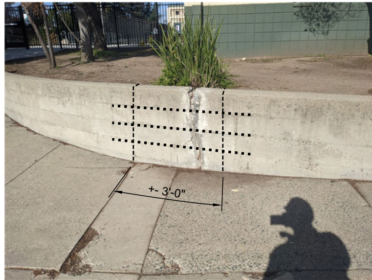
LOCATION: TOP OF RAMP AT AREA 5. REMOVE AND REPLACE (E) CURB. PROVIDE MIN. (3) #4 REBAR DOWELED IN 12" MIN. MATCH (E) FORMWORK FINISH.
